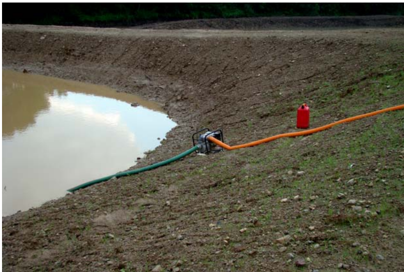
With each rain, I would pump water out of the creek side pond up into the large pond. This picture shows the height difference from the large pond to the outer creek pond and shows how much dirt was needed to build this huge pond dam.
