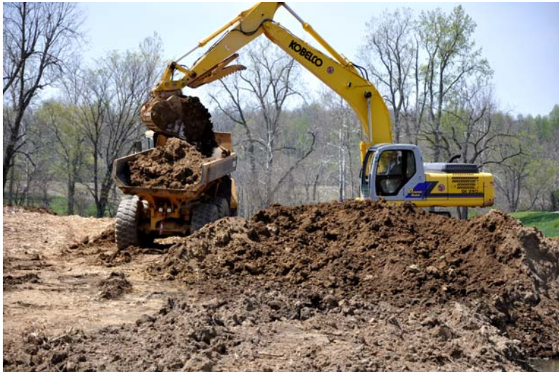
The off road trucks could pivot, so if they drove onto a edge and fail over, the bed and cab would just pivot and not break off. These huge trucks fail over twice while building the banks.
